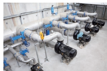
Sewage treatment plant
