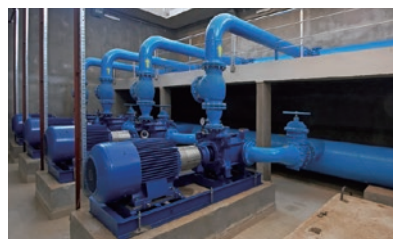
Building water pumps
