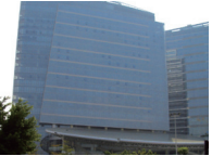
Guangzhou FA Center MITSUBISHI ELECTRIC AUTOMATION (CHINA)LTD.
