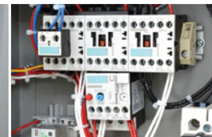
3 Contactor Bypass
