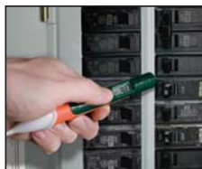
Non-contact InfraRed Temperature measurement
