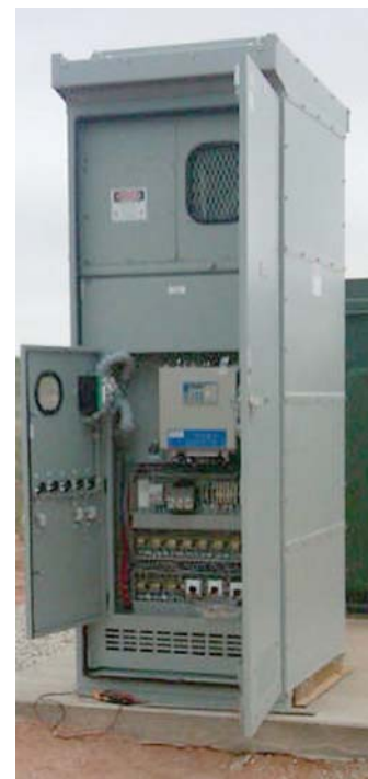
HRVS-DN in NEMA 3R special "outdoor" enclosure for harsh environments Figure 2
