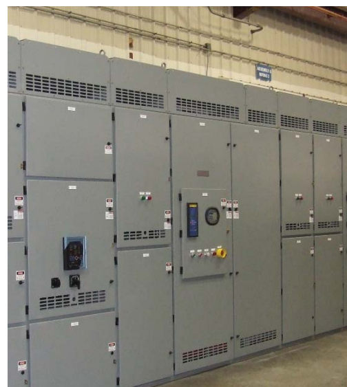
Metal-clad type construction
