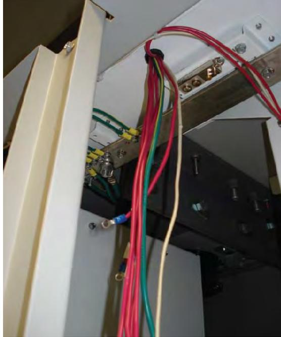
6. Route the control wires down through the grommeted cutout into the control power disconnect section ([Figure 34](#)).
