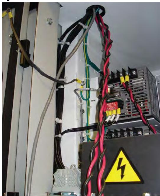
5. Route the 3-fan control wires, 2 cabinet over-temperature control wires down through the grommeted cutout into the center of the DC choke section ([Figure 33](#)).
